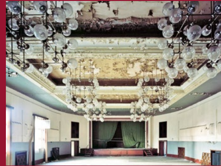
PHOTO: The hall prior to its refurbishment
