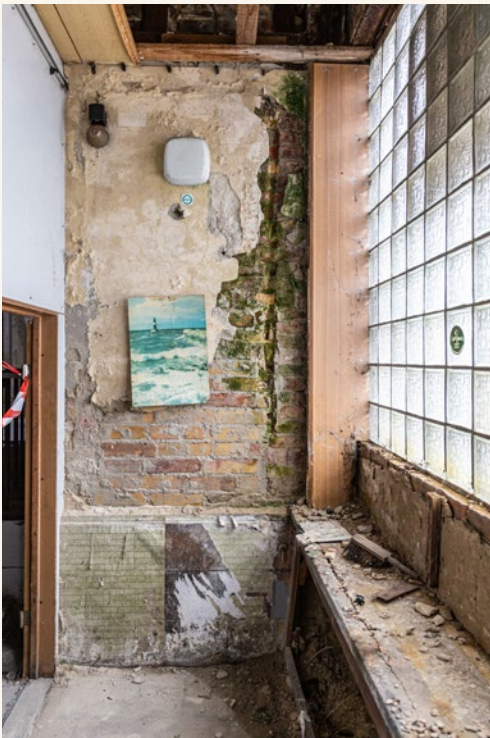
PHOTO: Entrance with cash register counter prior to refurbishment, 2023
