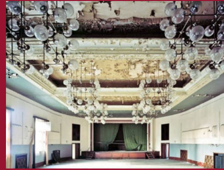
PHOTO: The hall prior to its refurbishment
